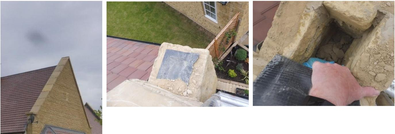
Images depict a raking parapet with stone copings. Various failings of the 3 lines of defence are present such as a horizontal DPC of incorrect width which lacks support across the cavity, a lack of mortar bedding across the full width of the wall and missing mechanical fixings leading detachment of the coping, and the omission of the cavity tray.
