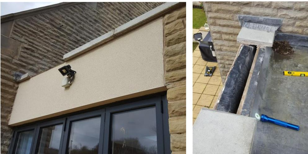
The cavity tray provision is the third and final line of defence in parapet construction. The failures range from poor cavity tray joint detailing, inadequate support and incorrect or lack of adequate provision for removal of trapped from the cavity.
